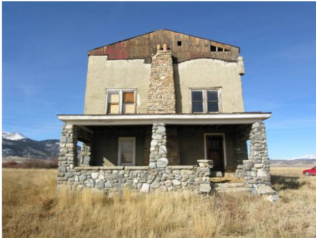
The main south entry stone porch, note the tapered corner columns and the deteriorated concrete ledge caps or sills in the openings.
