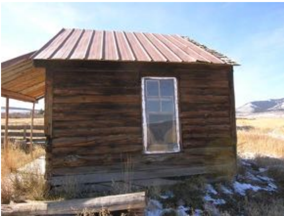
Cabin, east elevation, showing missing sash and plexiglass covering.
