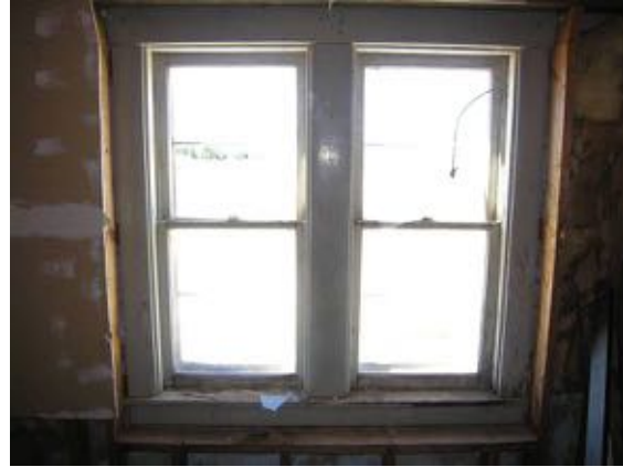
Windows, room #102, note painted finish. Note the furred out walls and unfinished drywall.
