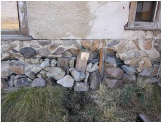
East elevation foundation veneer wall damage.
