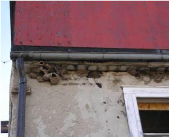
North edge of original roof deck with red painted plywood gable roof above. Note gutter and downspout from the flat roof that is no longer functional with the gable roof and the mud nests from Cliff Swallows under the gutter.
