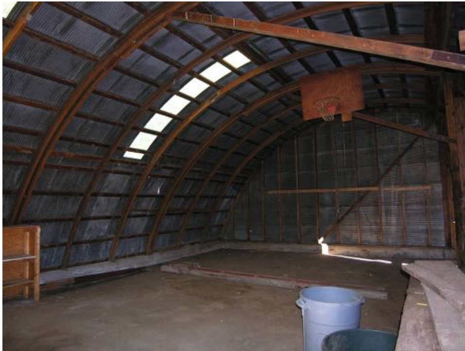
The Quonset has a series of arched laminates tied with wood battens. The end walls are studs.
