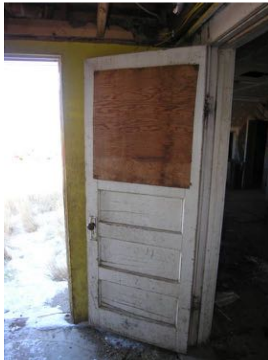
The exterior door within the north entry addition leading to the kitchen. Note the cracked wood panels and glass is missing. This was apparently the original entry door that was moved from the opening at the east end of the kitchen to this location at the west end of the kitchen, within the north entry addition.
