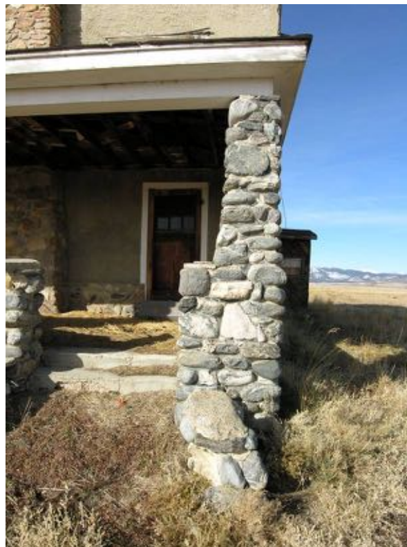
The main entry porch on the south elevation, the walls of the porch are generally structurally sound, but the concrete floor and steps are cracked and deteriorated.
