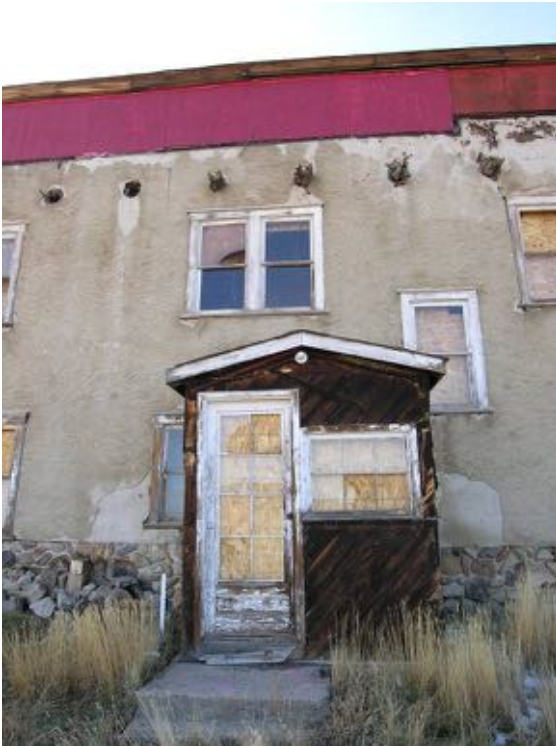
The east entry addition from the 1950s-1960s was never finished with siding or stucco and the original tar paper that was installed on the diagonal plank sheathing did not survive.
