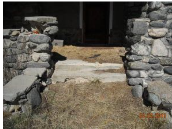
Stair to the south entry porch, note spalled and cracked concrete.
