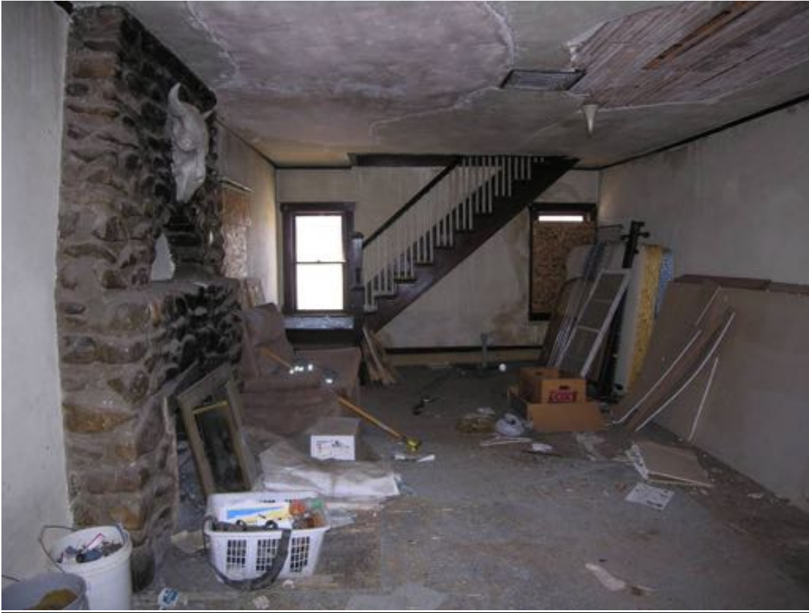
Interior view, first floor living room, view to the west. Note the deteriorated plaster lath ceiling, water damage on ceiling and walls, the original stone fireplace, the strip tongue and groove pine/fir flooring, and stairway leading to the second floor.
