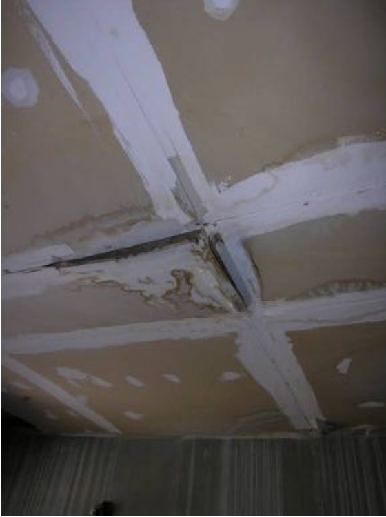
Second floor ceiling showing water damage.
