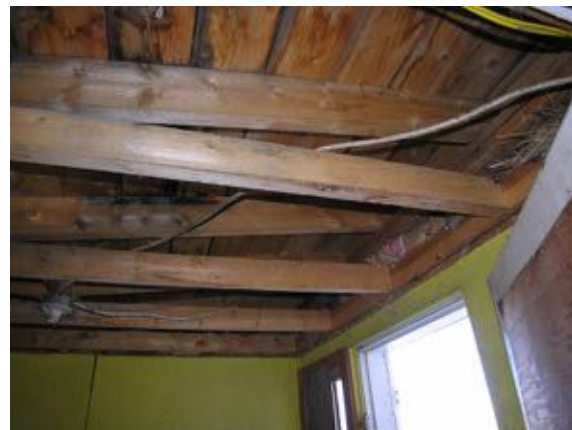
The north entry/utility addition, showing the roof framing system.
