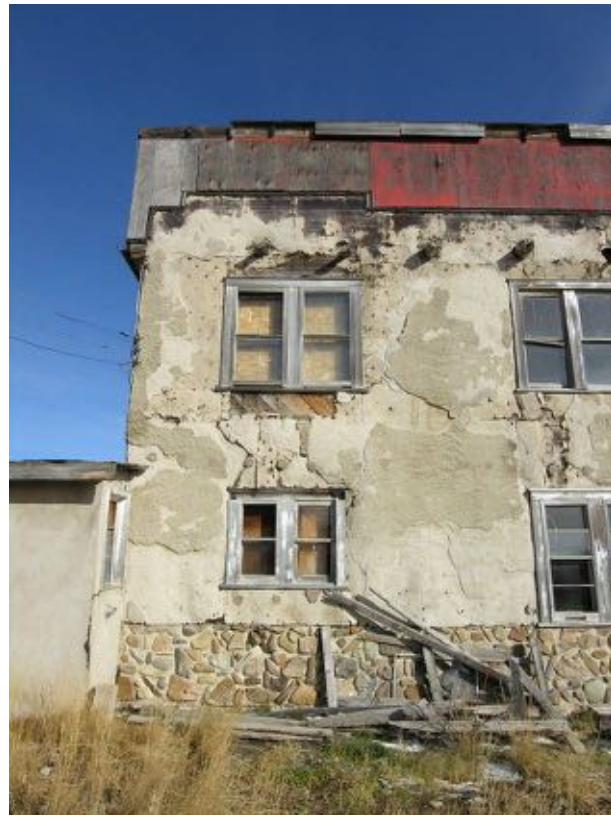
Exterior of the west wall, note the exposed diagonal wood plank sheathing where the stucco has failed.
