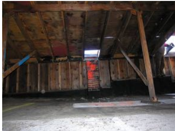
The brick chimney/flue on the west side of the original roof.
