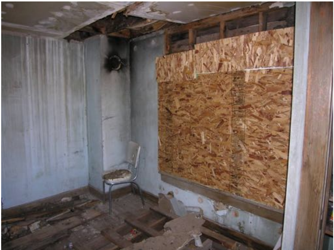
Room 204, Bedroom, the 2nd floor ceiling joists are visible through the gap in the plaster ceiling and the wall framing is visible above the OSB panels on the windows.
