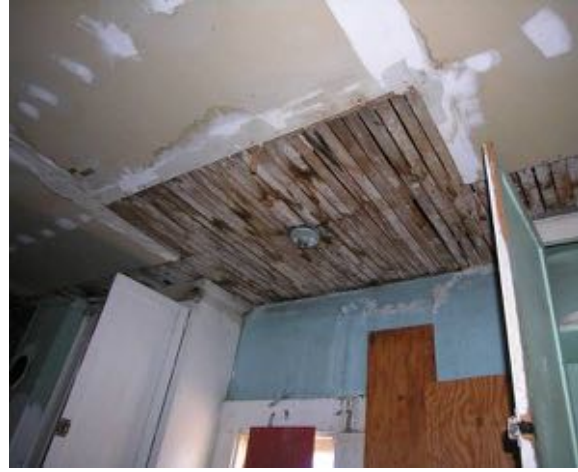
Interior, kitchen, room #105, view to the west. Note the exposed wood lath under the sheetrock and the painted kitchen cabinets.
