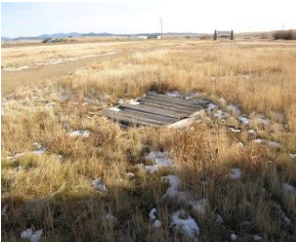
The well cover is wood planking set on the ground above the well and vulnerable to deterioration or a vehicle inadvertently driving over it in the winter.
