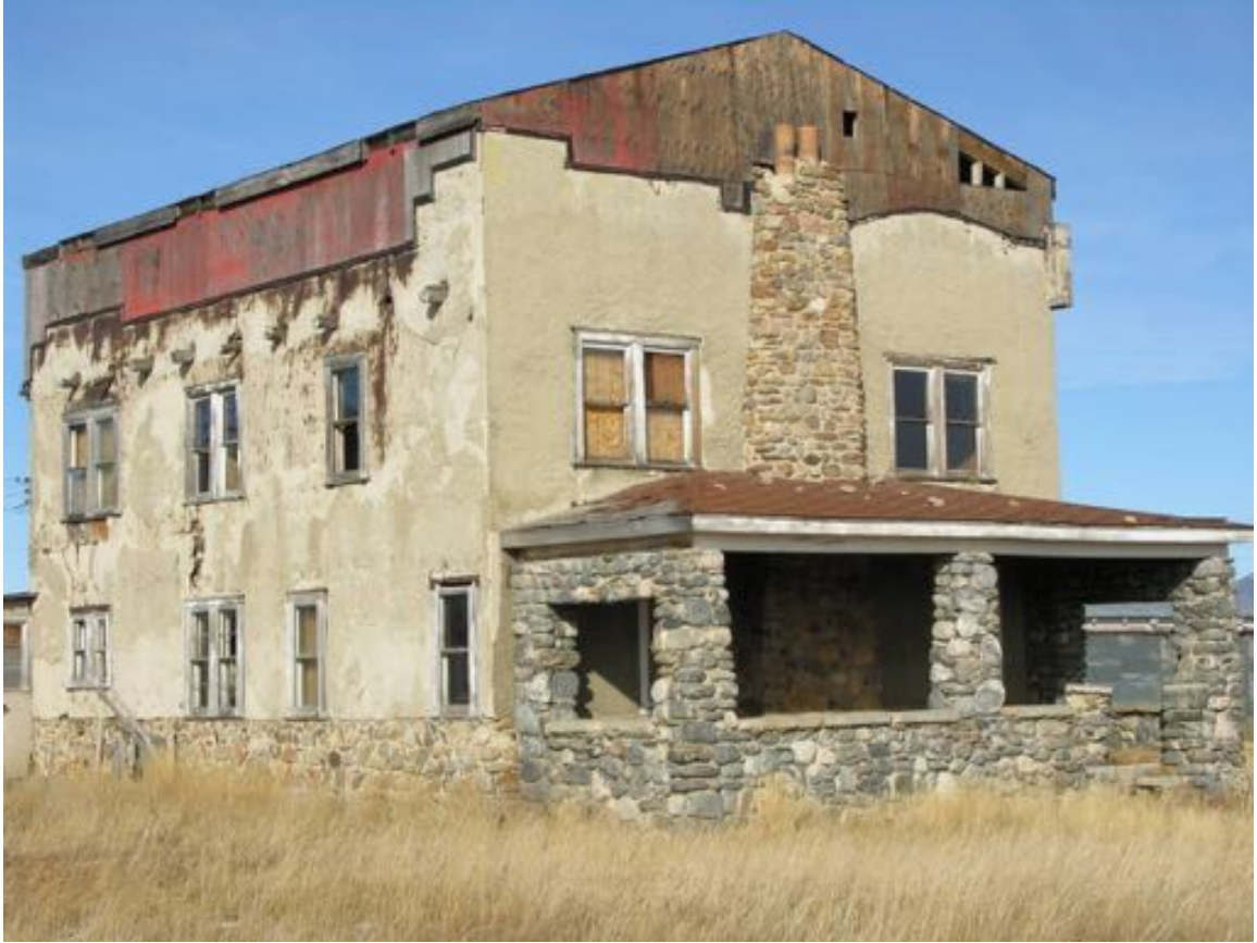
The south and west elevations of the Cline main ranch house, showing the original 1/1 double hung wood windows that are often paired, note that while the glass is broken or missing on many of the windows, the wood sash is intact.
