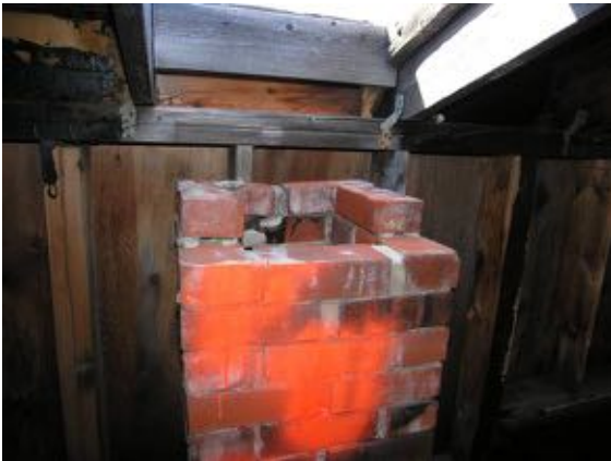
The brick chimney/flue on the west side of the original roof, note the upper courses of brick are missing and the mortar is crumbled at the top.
