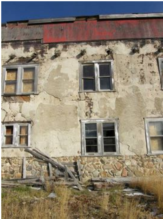
The heavily deteriorated stucco on the west elevation, exposing the wood sheathing in places on the walls. Also note the rotted or missing vigas (log ends).
