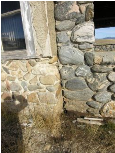
Southwest corner of the house at the joint with the south entry porch, note the differences in the masonry types. Also note the concrete footing and stone masonry veneer wall of the house foundation.
