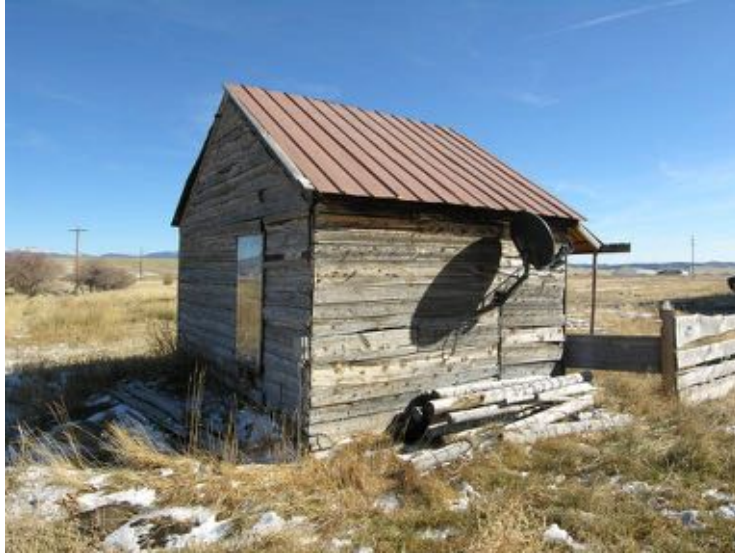
The Cabin, west elevation. The siding appears installed without adequate weather sealing.
