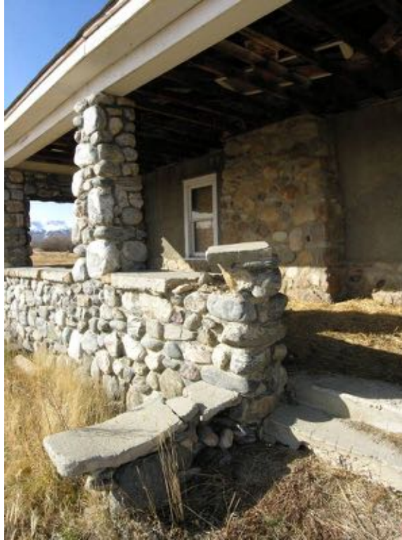
The main entry porch on the south elevation, the walls of the porch are structurally sound, but the concrete floor and steps are cracked and deteriorated.
