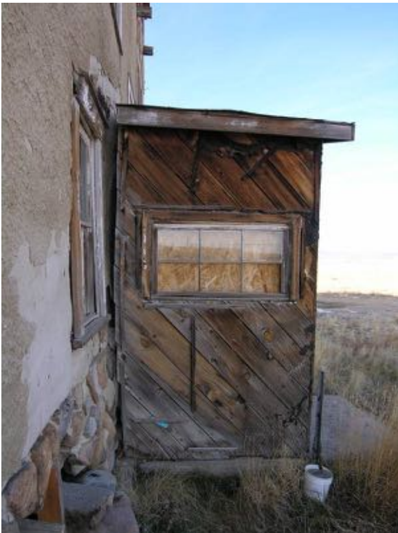
Separation of the entry vestibule on the east elevation of the building.
