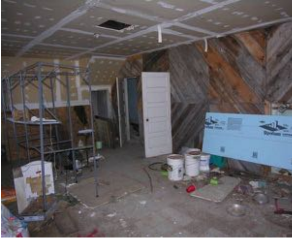
Interior, kitchen, room #105, view to the southeast. Note the barn wood on the wall and the unfinished sheetrock on the ceiling and east wall.
