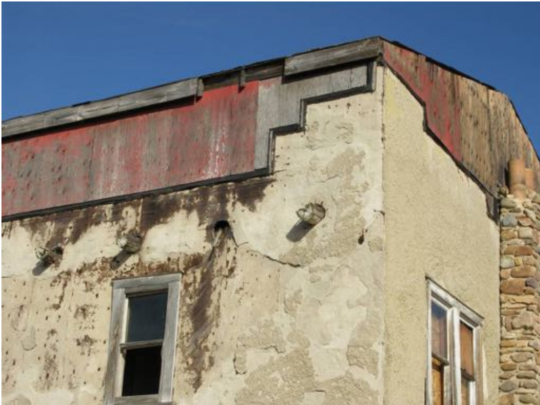
Overframed gable roof built on the parapets, rotted vigas and deteriorated stucco at the southwest corner of the house.
