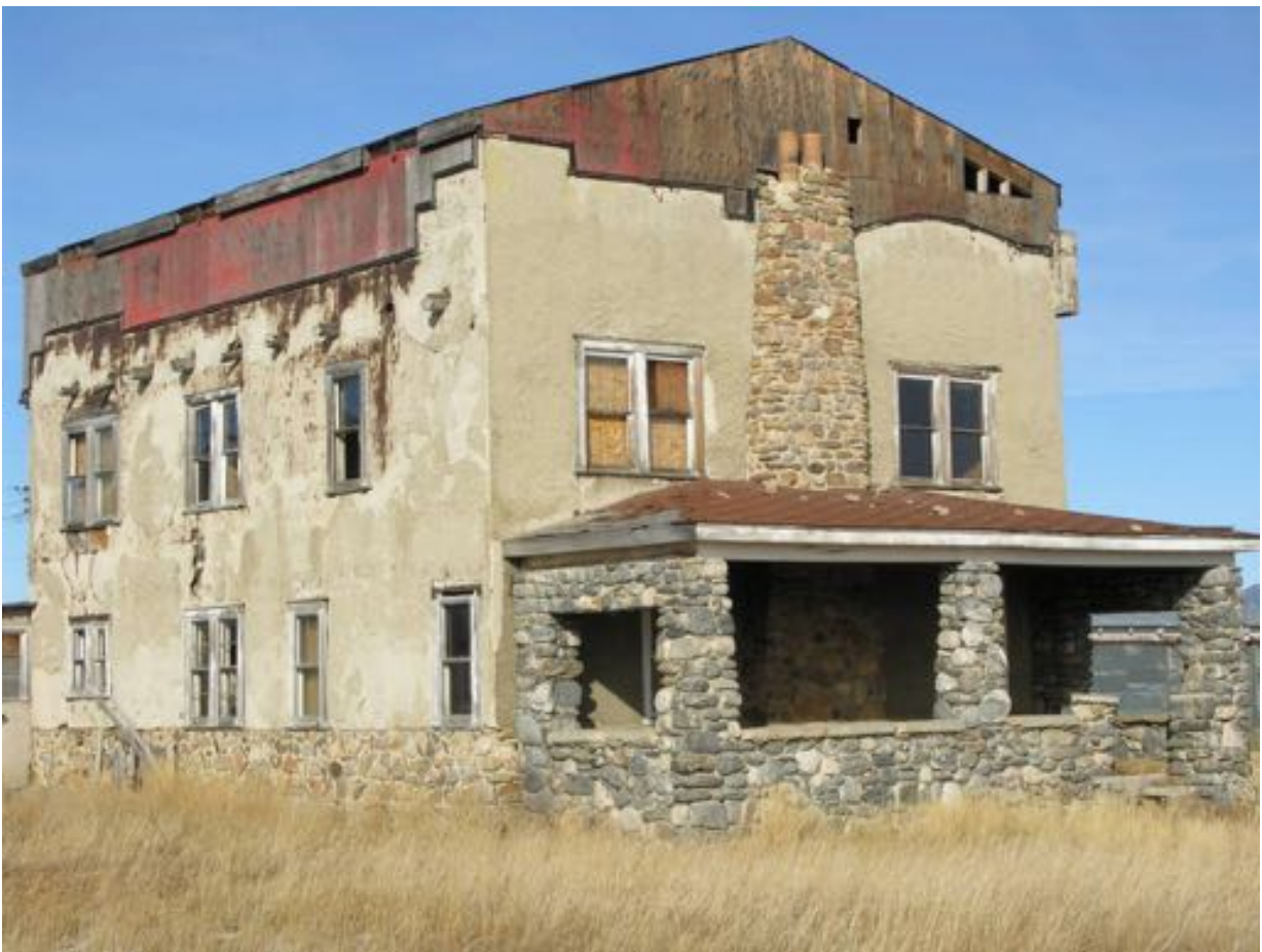
The Cline main ranch house, view from the southwest, showing the deteriorated stucco system on the west elevation, including rotted vigas, the stone veneer applied at the base of the west elevation, and the stone main south entry porch.
