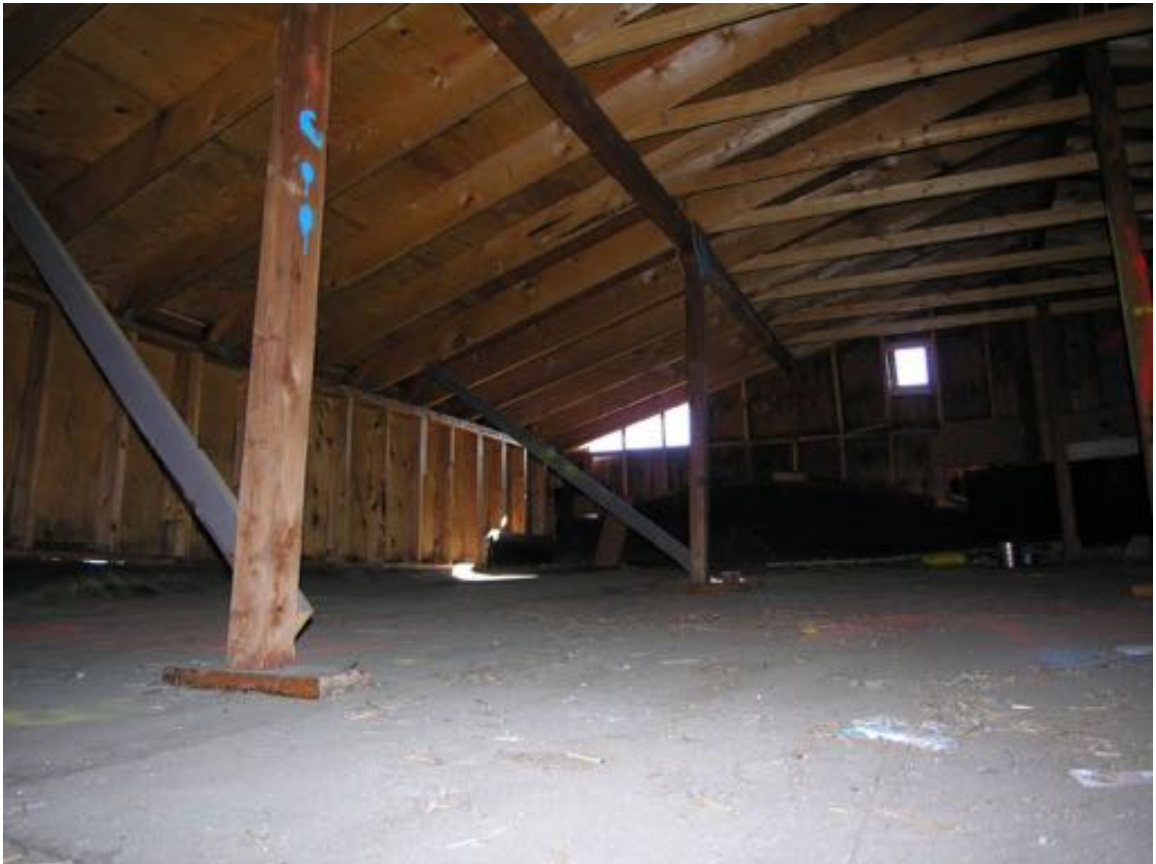
The modern gabled roof system, built over the original flat roof, looking toward the southeast.
