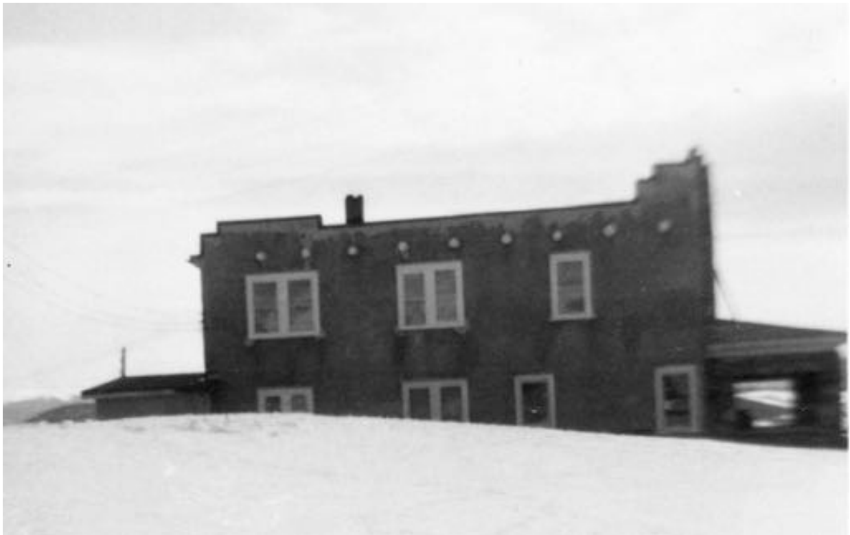
Historic Photo #3 undated, but it is c.1950s/1960s, view of the west elevation. note the original roof line, and the 1/1 double hung wood windows.
