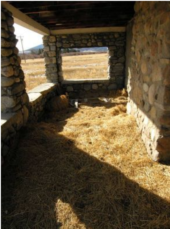
The main entry porch on the south elevation, view to the west; note the spalled and eroded concrete sills or ledge caps. The heavy layer of hay/straw made it impossible to evaluate the entire concrete floor.
