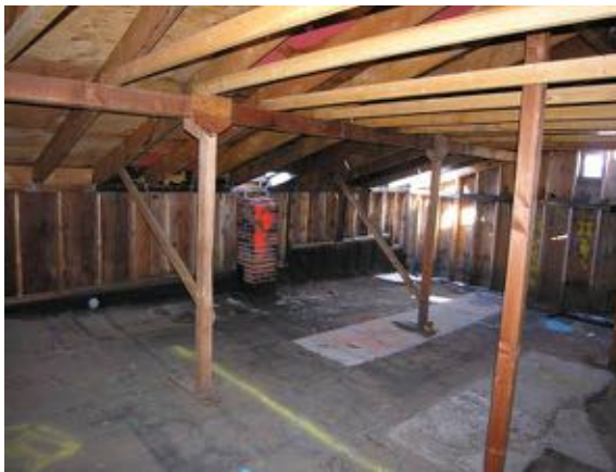
Original roof deck and parapets, over framed with modern gable roof, view to the northwest corner.
