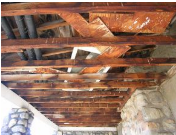
The roof system of the south end porch, showing the exposed light framing of the rafters.
