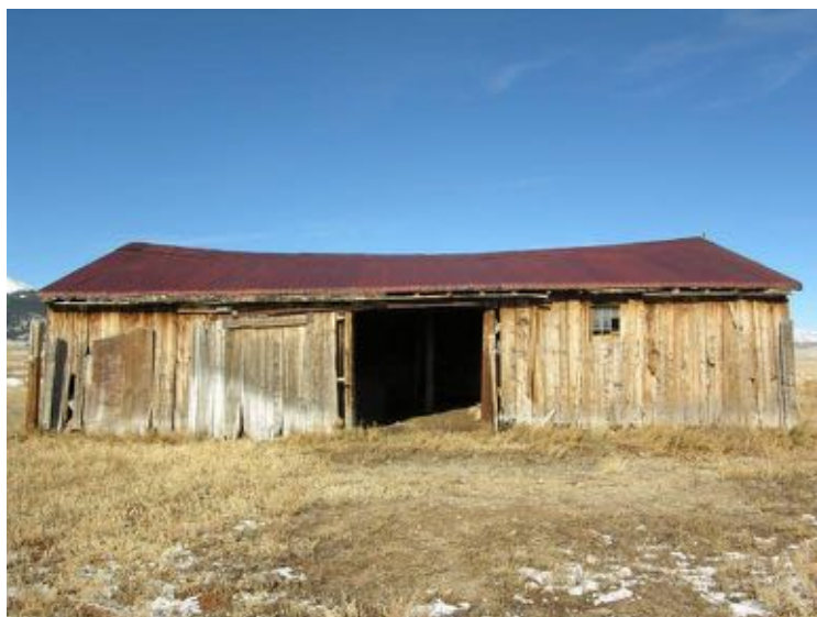
The Barn is roofed with unpainted corrugated sheet metal.
