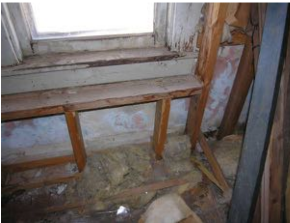
Interior room #102, view to the west. Note the 2”x4” furring over the wood lath and plaster.
