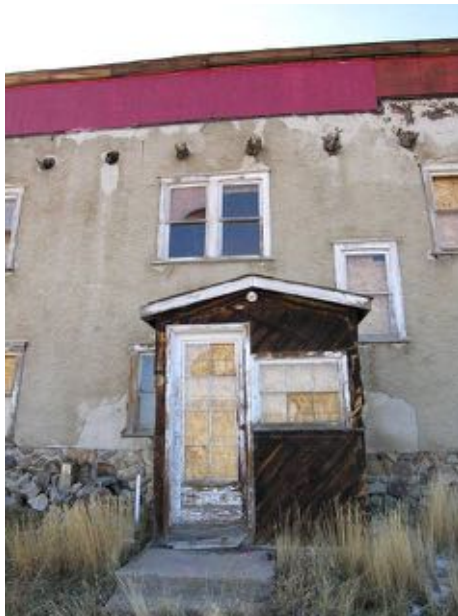
East entry addition built in 1950s -1960s and the construction was never finished. The opening through the exterior wall of the house into room #107 was a window originally, not a door.
