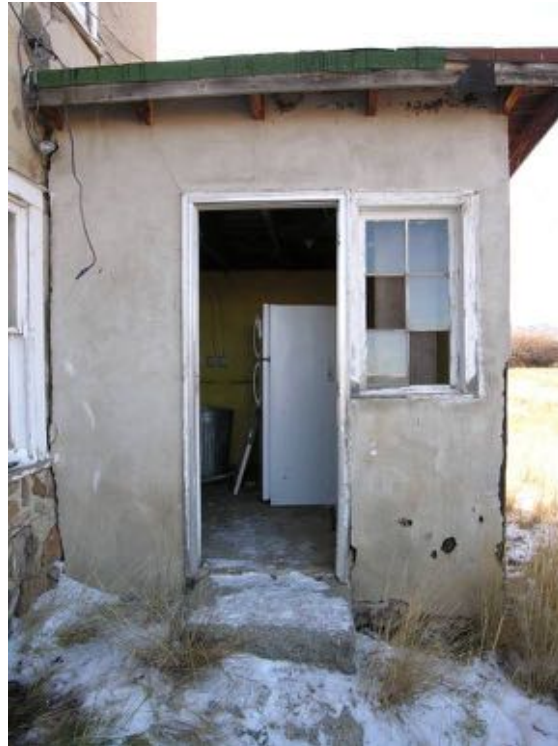
The north entry addition from the 1950s -1960s replaced an earlier detached coal shed. This stuccoed addition was built when the door on the north elevation was moved from the original location on the north wall to the other side, inside this shed.
