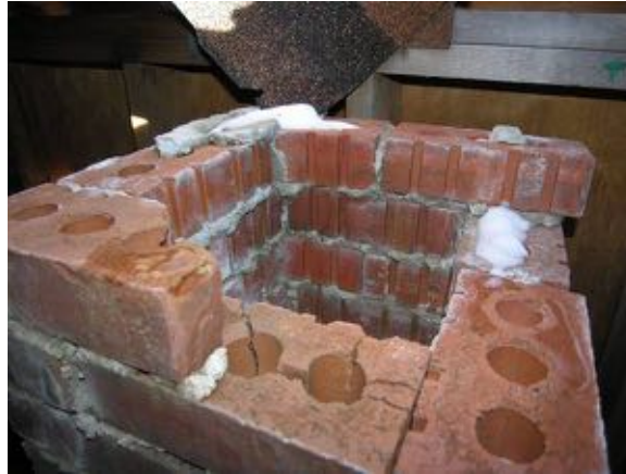
Detail of the brick chimney/flue on the east side of the original roof, now covered by the gable roof.
