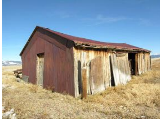
The Barn, viewed to the north west. The south elevation is wood and clearly deteriorated. The west elevation is sheathed over in sheet metal.
