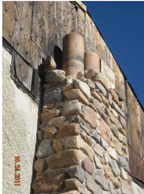
Deteriorated stonework and eroded mortar at the top of the historic south chimney cap.
