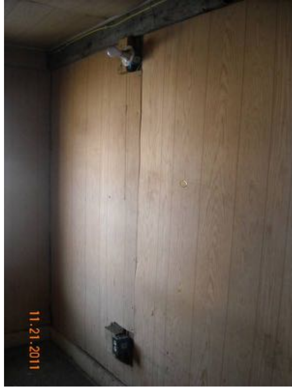
Cabin electrical wiring showing unsafe wiring exposure.
