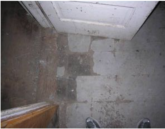
Remnants of a tile on the kitchen floor. Note the wood strip flooring underneath.
