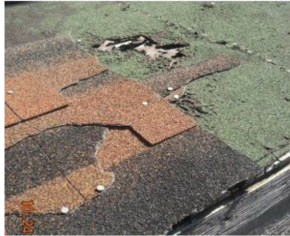
Deteriorated asphalt roofing layers on the north entry addition, note that the green roll roofing is the earliest layer, dating from the construction of the addition in the 1950s -1960s.
