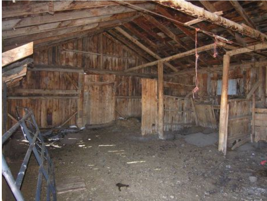
The Barn has steel rod collar ties that appear inadequate to maintain the building shape.
