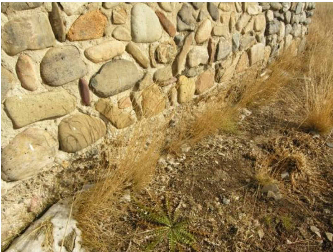
Foundation of the main ranch house with a spalled and eroded concrete footer and a rock masonry veneer wall above.
