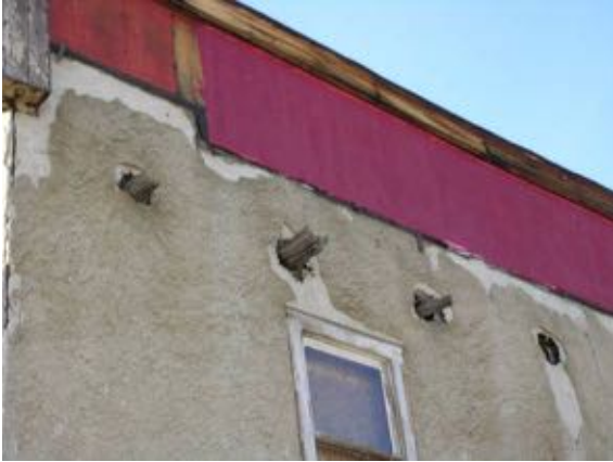
The rotted and missing log vigas on the east elevation, these are not structural.
