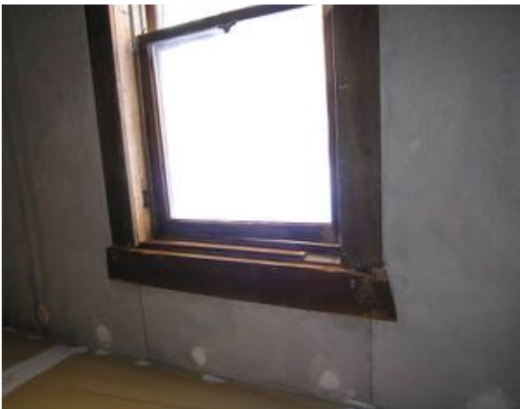
Southwest stair window, note stained and varnished finish on the window and casing. Also note the drilled holes that were patched after an insulation project in recent years, apparently.
