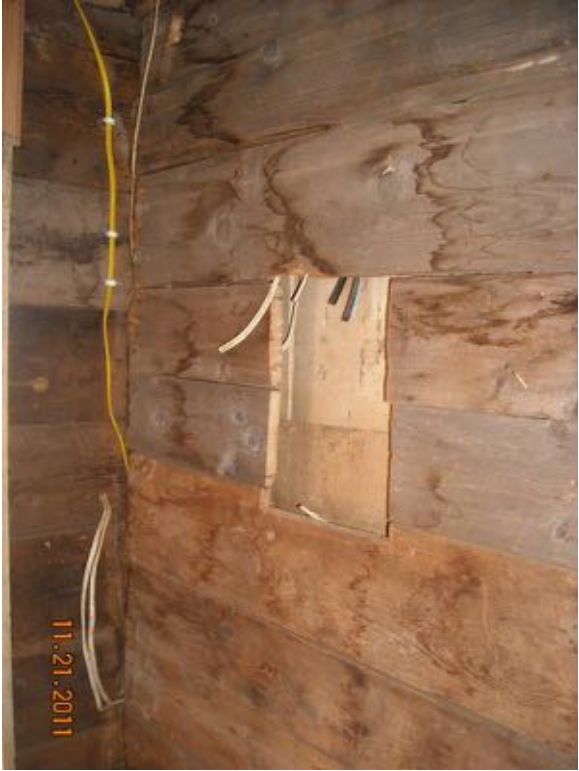
Cabin unsafe surface wiring and apparent former location of electrical breaker panel and shutoff.
