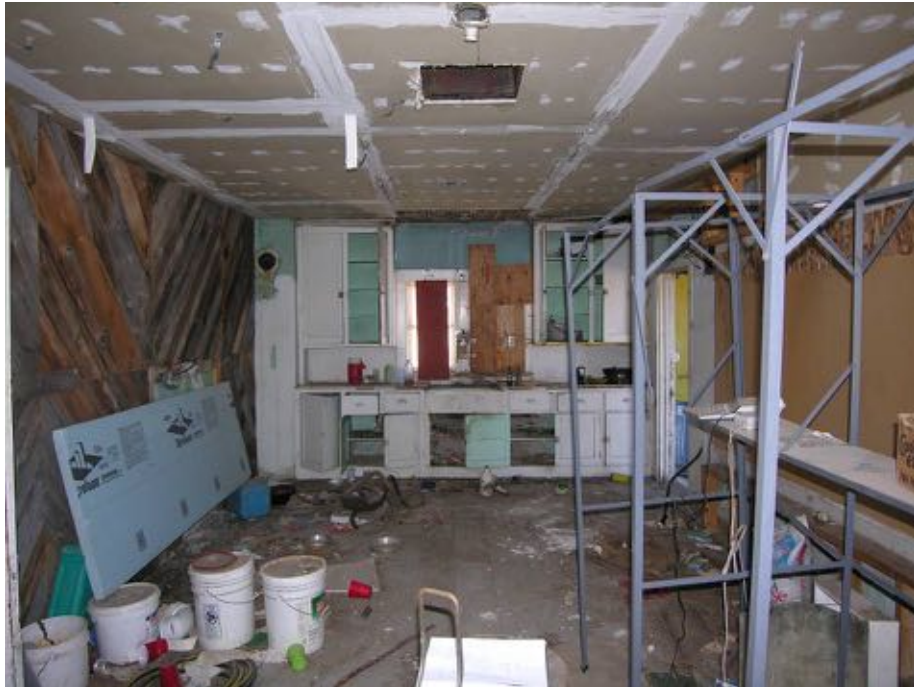
The first floor kitchen, looking to the west. Note the paper-covered gypsum board ceiling, the rough barnwood wall covering, and the original built-in cabinetry. The floor tiles are largely obscured by litter and dirt.
