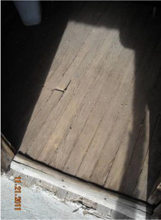
Strip tongue and groove flooring of the Cabin. Note the inadequate entry threshold.
