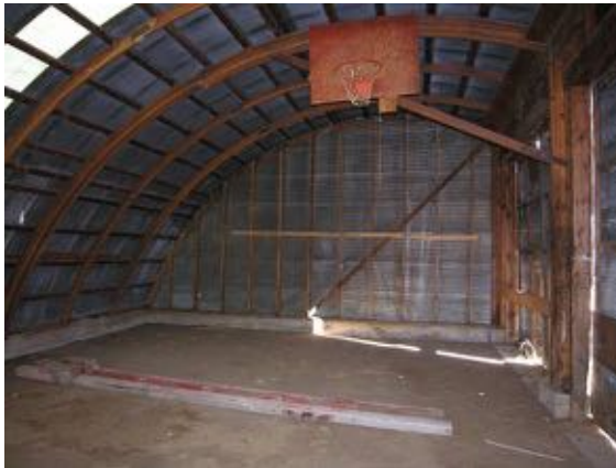
The concrete footer for the Quonset is clearly evident.
