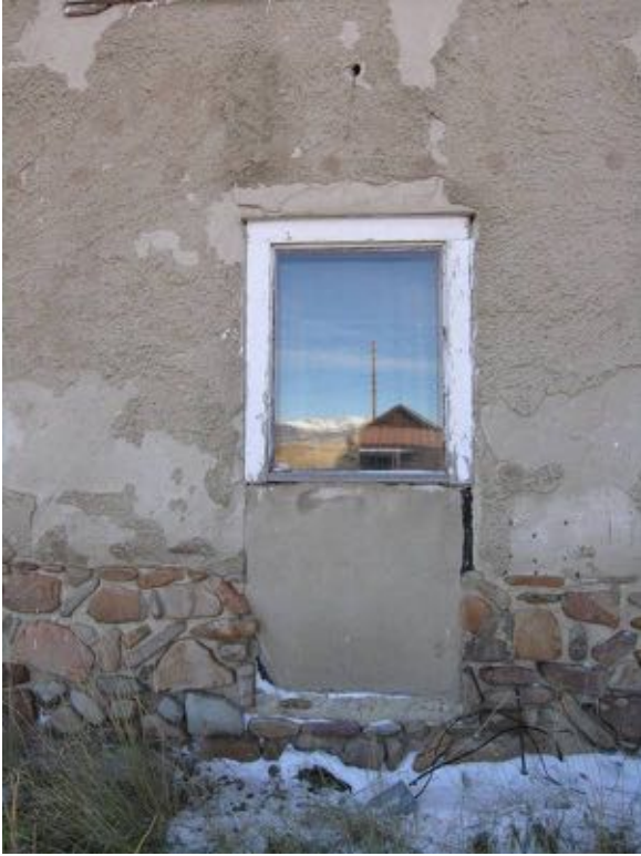
North elevation, east end, this half window is in the original door opening that led to the kitchen.
