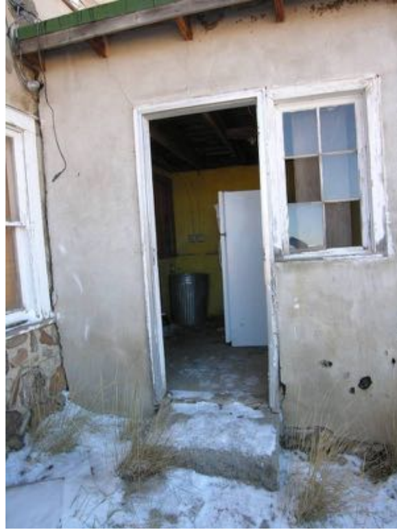
North entry addition. Note that the door is missing, but it is apparently stacked inside the kitchen. Note the broken glass in the window.
