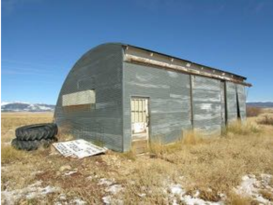
Quonset, south elevation. Corrugated metal material covers the frame below.
