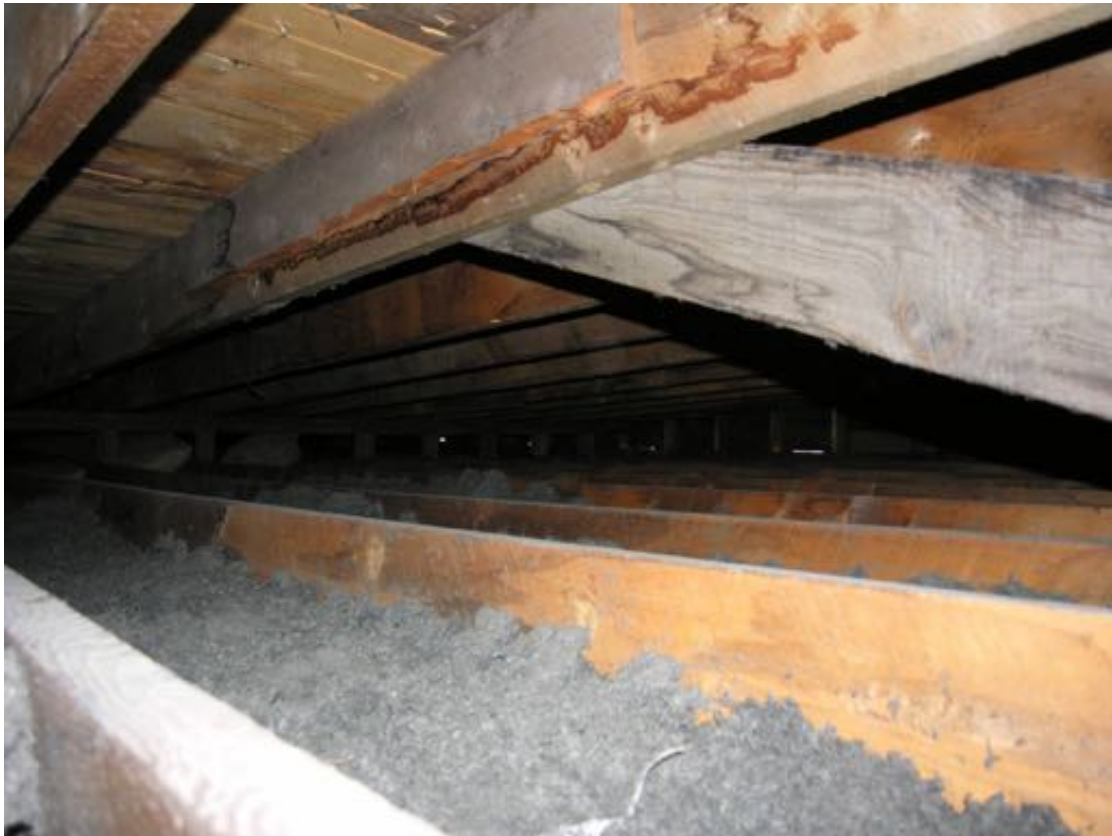
Loose fill insulation between the ceiling rafters above the second floor of the house.
