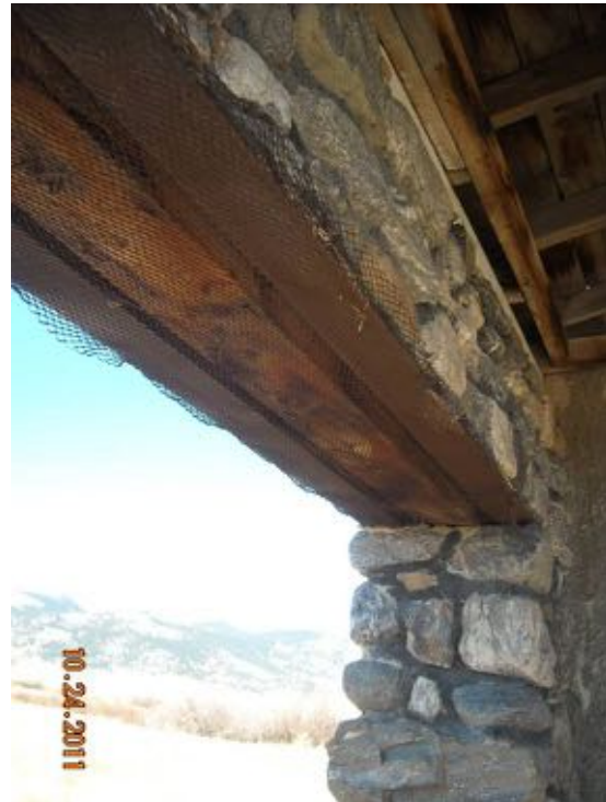
Header detail of the main entry porch, west end, on the south elevation; note the wood and wire mesh evidently intended to support stucco.
