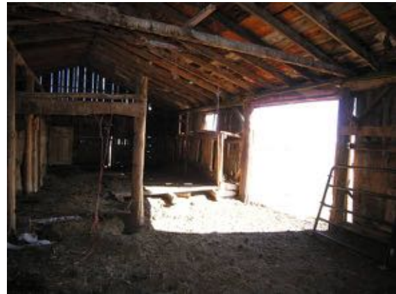
The Barn is constructed pole barn style, with vertical foundation posts.
