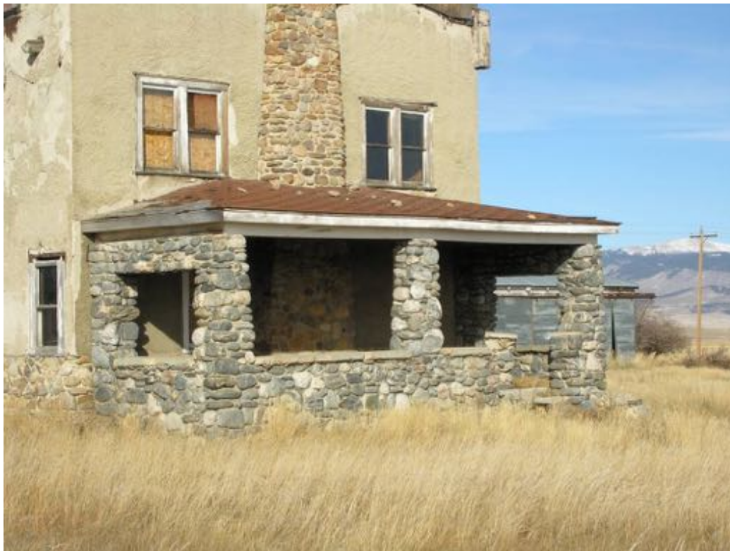
The hipped roof of the main south entry porch shows deteriorated and missing asphalt shingles.
