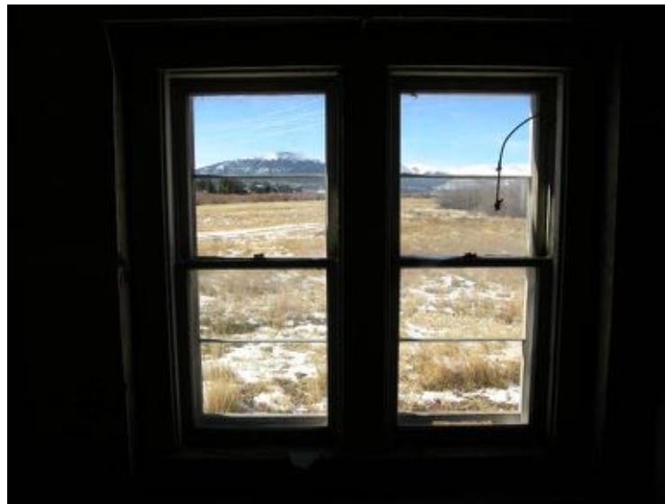
View to the west from the Main ranch house 1st floor bedroom. Note that the sash rope is detached.
