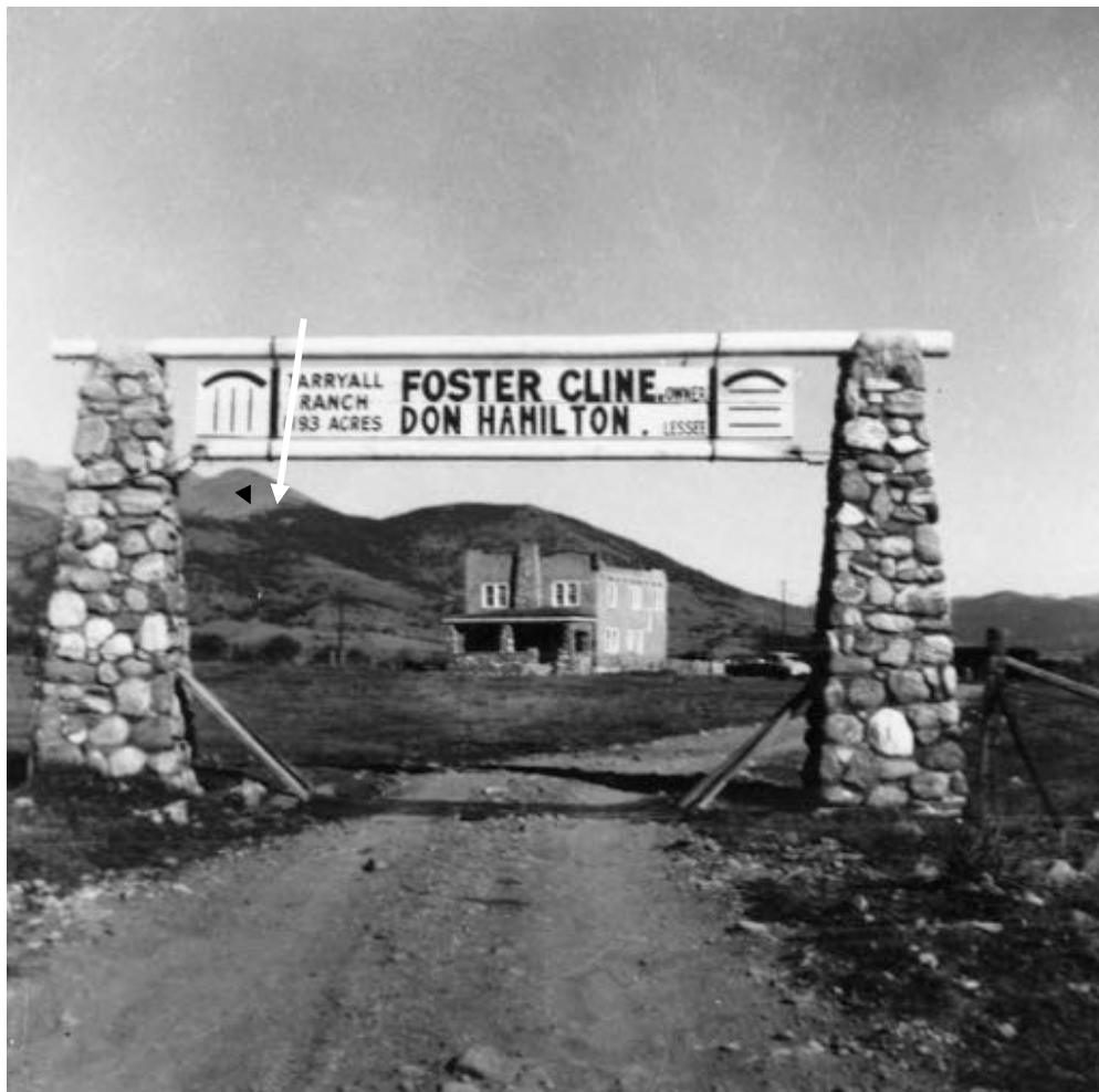
Historic photo #1, undated, but it is from the early 1950s according to Twila Brompton, daughter of Don Hamilton. The east and south elevations of the main ranch house seen through the gate posts. Note that the parapeted roof is in original condition without the current gable roof overlay and also note that the currently existing door and small entry addition on the east elevation do not exist in this photo, indicating that these are later alterations. An original window on the east elevation was later changed to a door.
