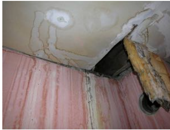
Water damage in a second floor bedroom ceiling. Note that the ceiling material is an added layer of paper-sided gypsum board.
