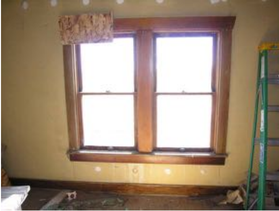
Windows, room #201, note stained and varnish finish as well as the baseboard. Note the drilled patched, holes from insulation work.
