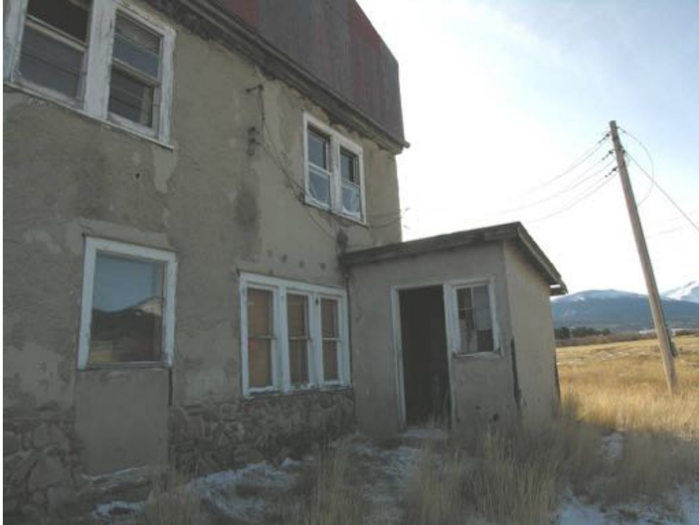
The north elevation, showing incoming electric service to conduit tubes of uncertain integrity.
