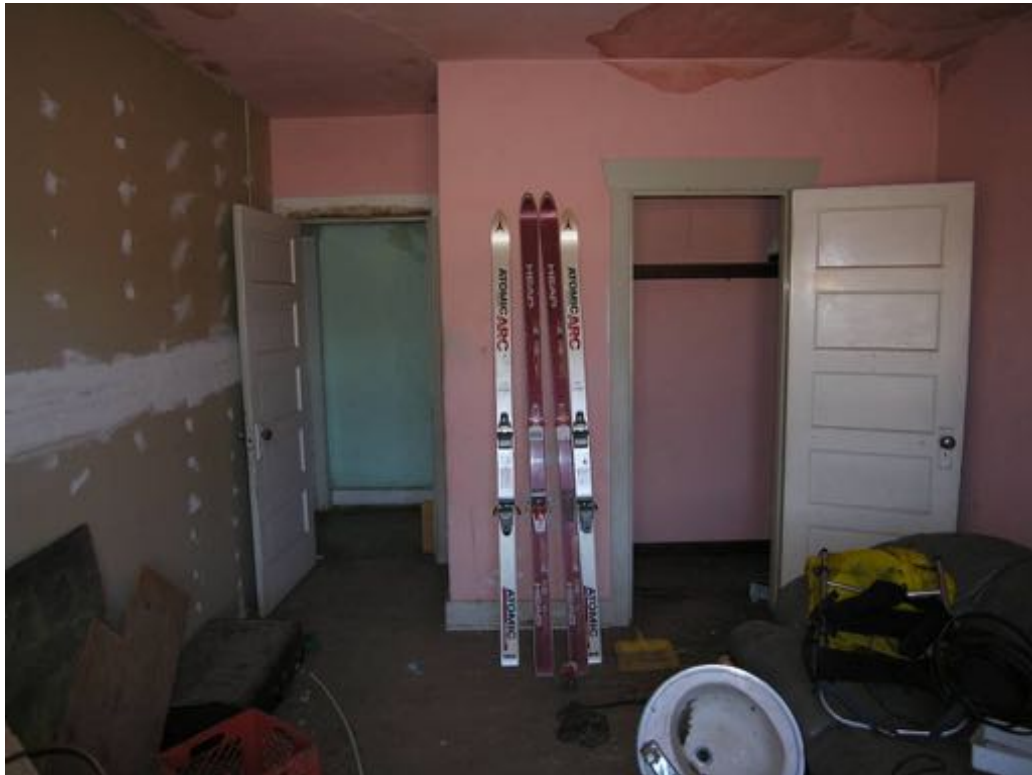
First floor Bedroom #102, view facing east. Note that the room has its original wood flooring and the walls and ceiling are original, but two walls have been furred out and covered with sheet rock that is only partially finished. The woodwork is original, but the stained and varnished finish has been painted.
