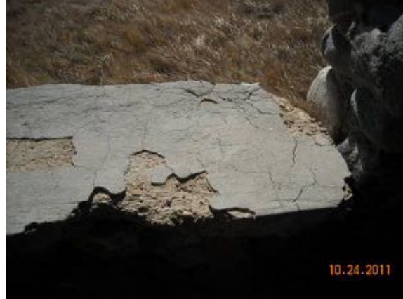
The spalled and eroded concrete “sills” or ledge caps on the main south porch.
