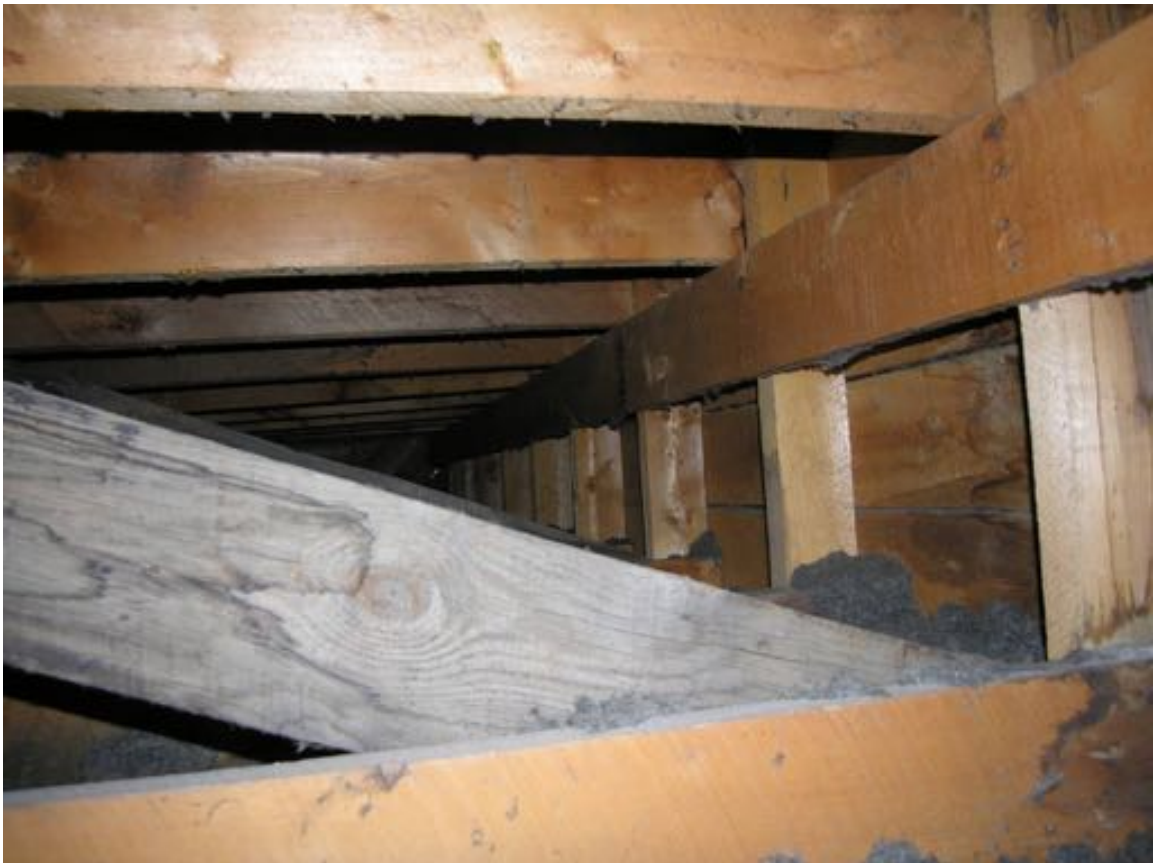
The original slightly sloped flat roof rafters (at the top of the photo) above the ceiling joists (foreground) for the second floor (diagonal is bracing), view at the south end of the roof structure.
