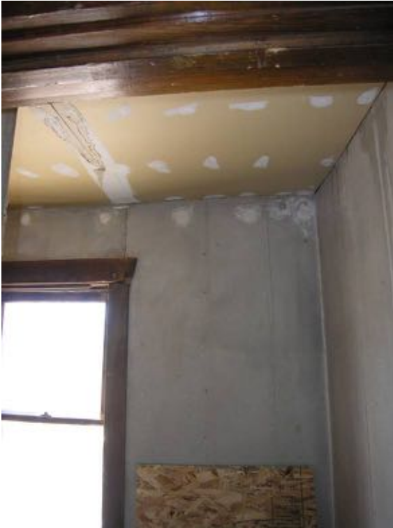
Southwest stair, view to the west. Note the unfinished drywall on the ceiling and patched holes in the wall from insulation installation.
