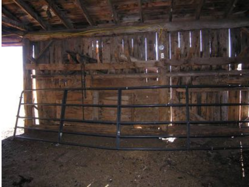
The Barn, showing surface mounted Romex wiring.
