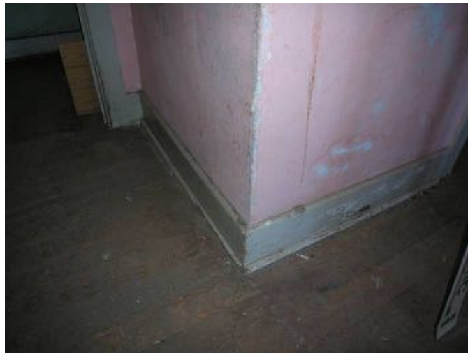
Second floor detail, showing strip flooring and painted baseboard.
