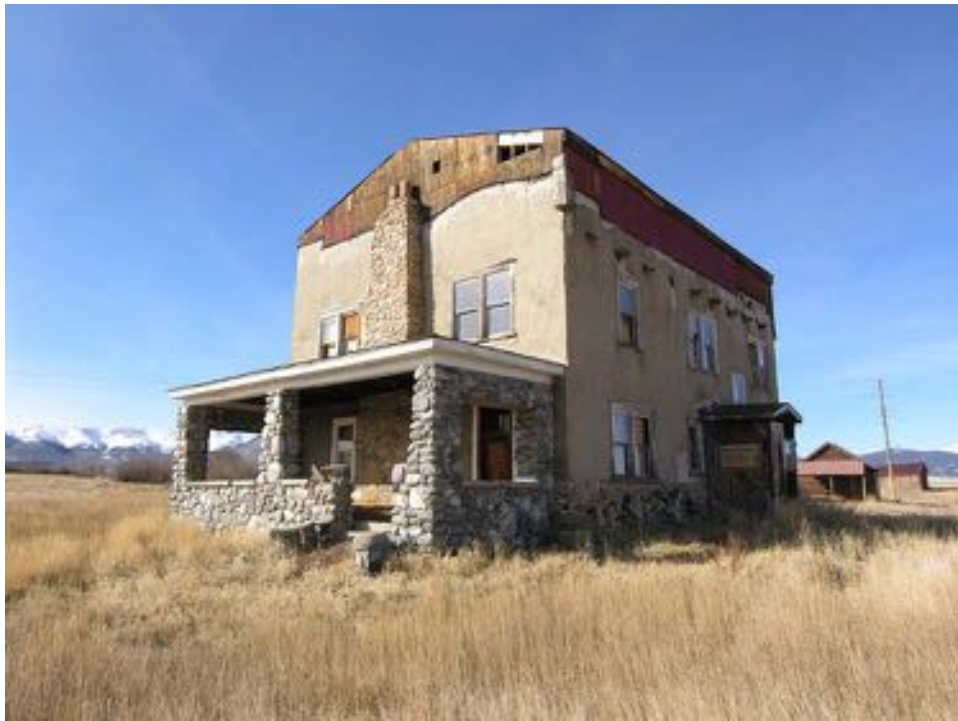
South and east elevations. Note the asymmetrical shaped original parapet with the overframed non-historic 1980s gable roof. There are also differences in the rustic stonework of the chimney and the
