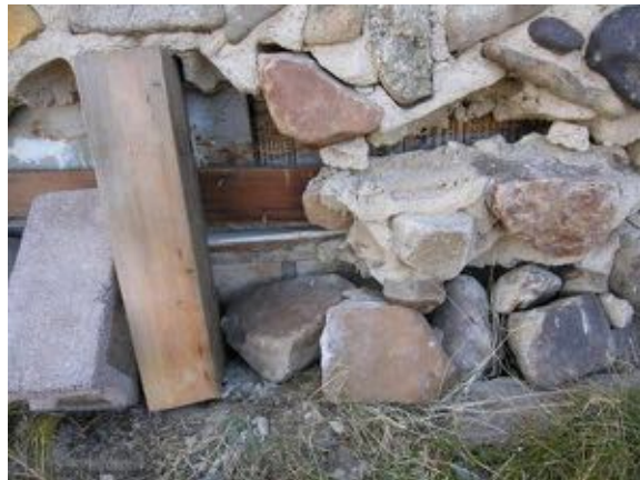
East elevation foundation veneer wall damage.
