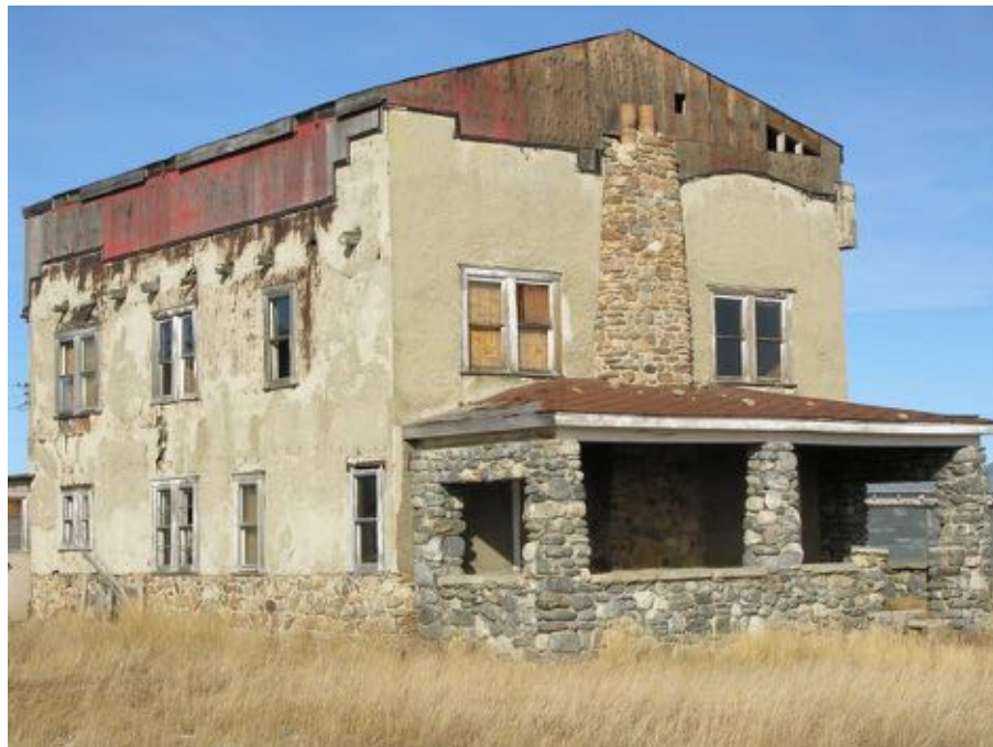
South and west elevations. Note the stucco and stone wall surfaces and the projecting vigas. The overframed roof was added in the 1980s, but the original stepped and curved parapet line is original and
