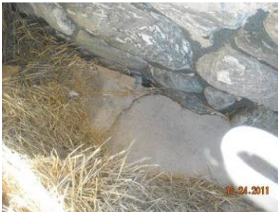
South entry porch concrete floor, note cracking.
