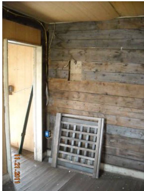
The back room of the Cabin, showing rough plank walls, beadboard ceiling, and strip tongue and groove flooring.
