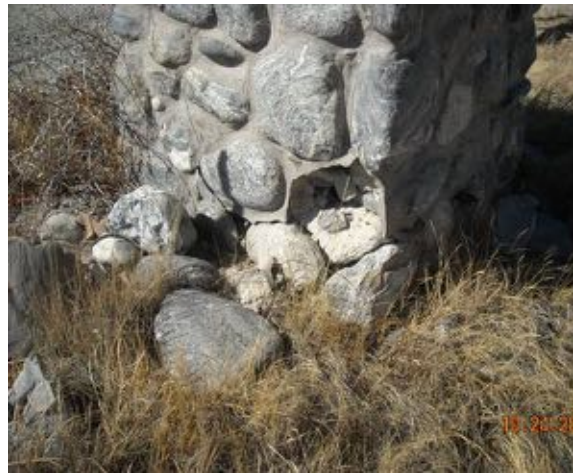
The stone work of the gate posts has deteriorated and needs repair to carefully match the original mortar, tooling and setting.
