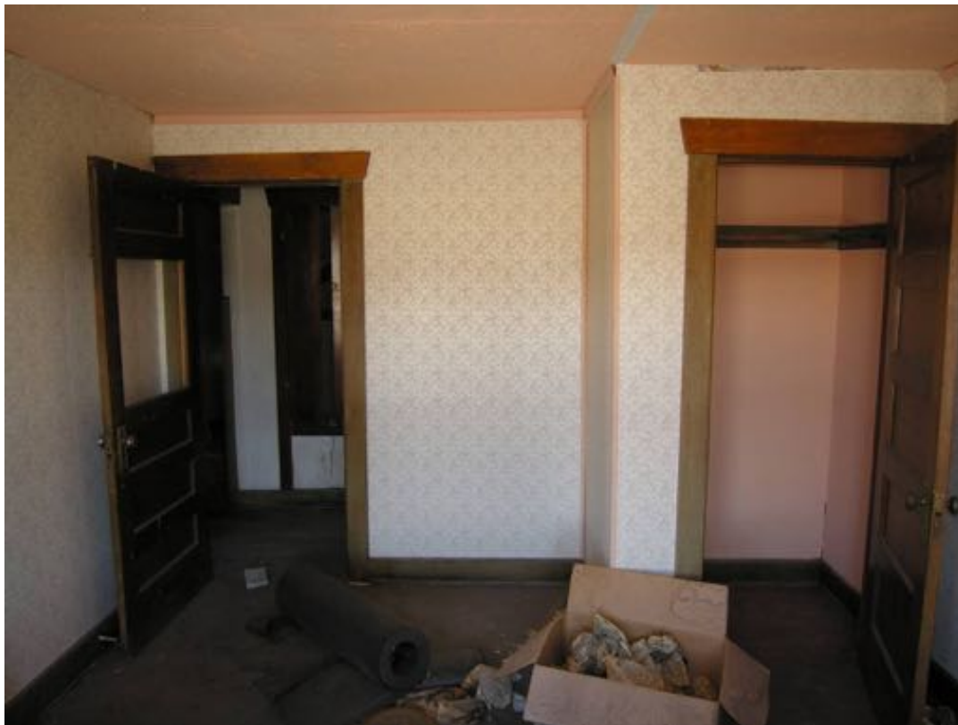
Bedroom, room 202, view to the east. Note the original flooring, walls, ceiling and woodwork – baseboards, casings and a small cornice molding. The doors are in place with their original hardware, but the door to the hall has had two panels removed and needs to be restored.
