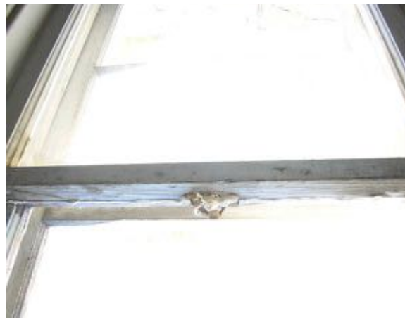
Windows, room #205, note deteriorated paint and the brass sash latch.
