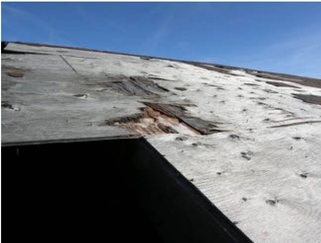
Large areas of the modern gable roof are missing shingles and in this case includes a major hole.
