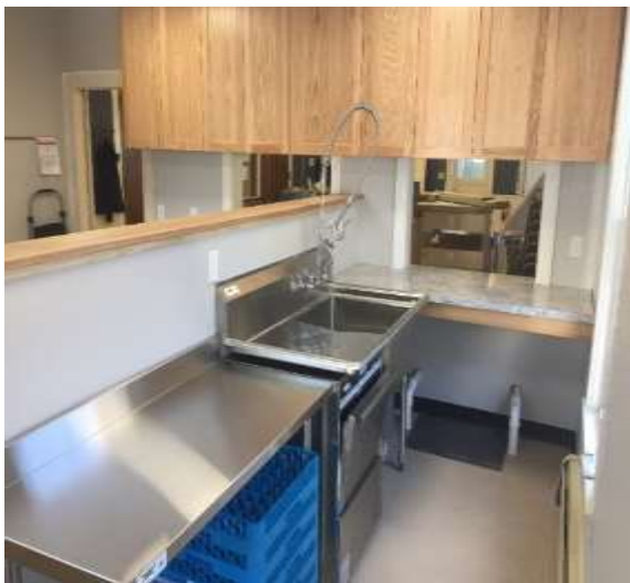
There are now two windows into the vestry area. This one is where the dishes are returned and can be rinsed and loaded into the NEW DISHWASHER! The one on the other side of the half wall is where the food goes out from the kitchen.
