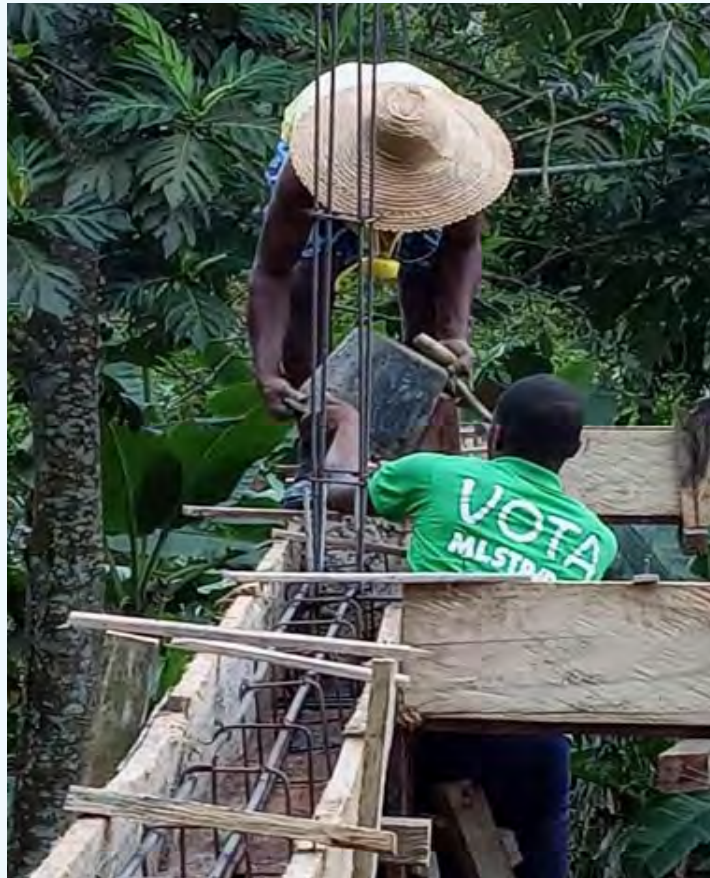
Filling The Concrete Structural Beams
