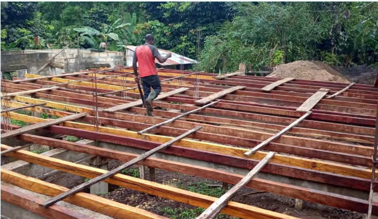
Floor Beams In Place
