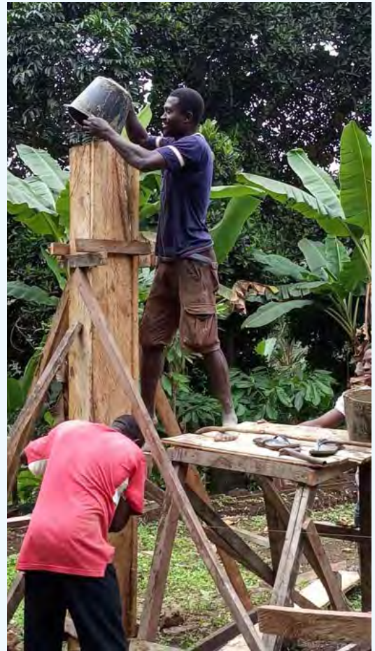
Digging, Setting and Filling The Concrete Pillars
