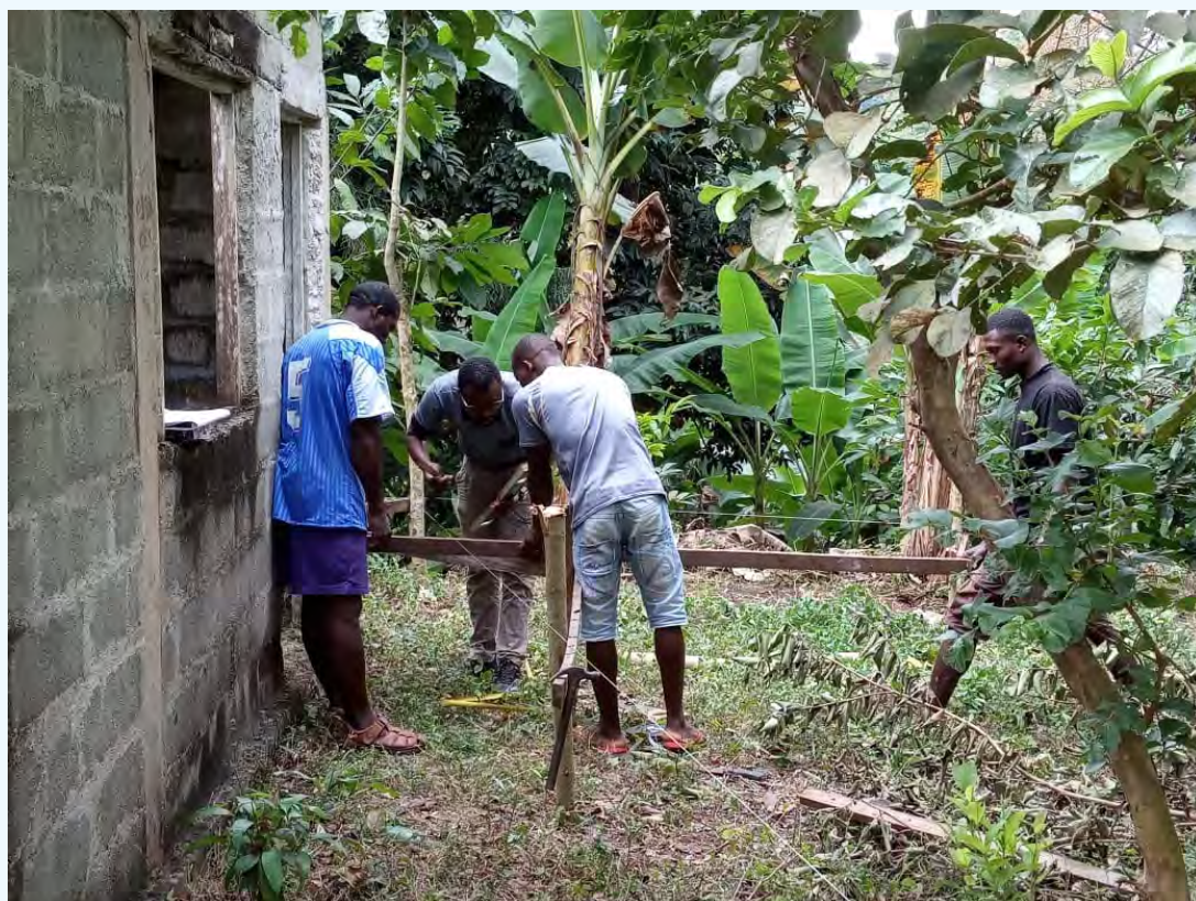
Measuring And Marking House Layout
