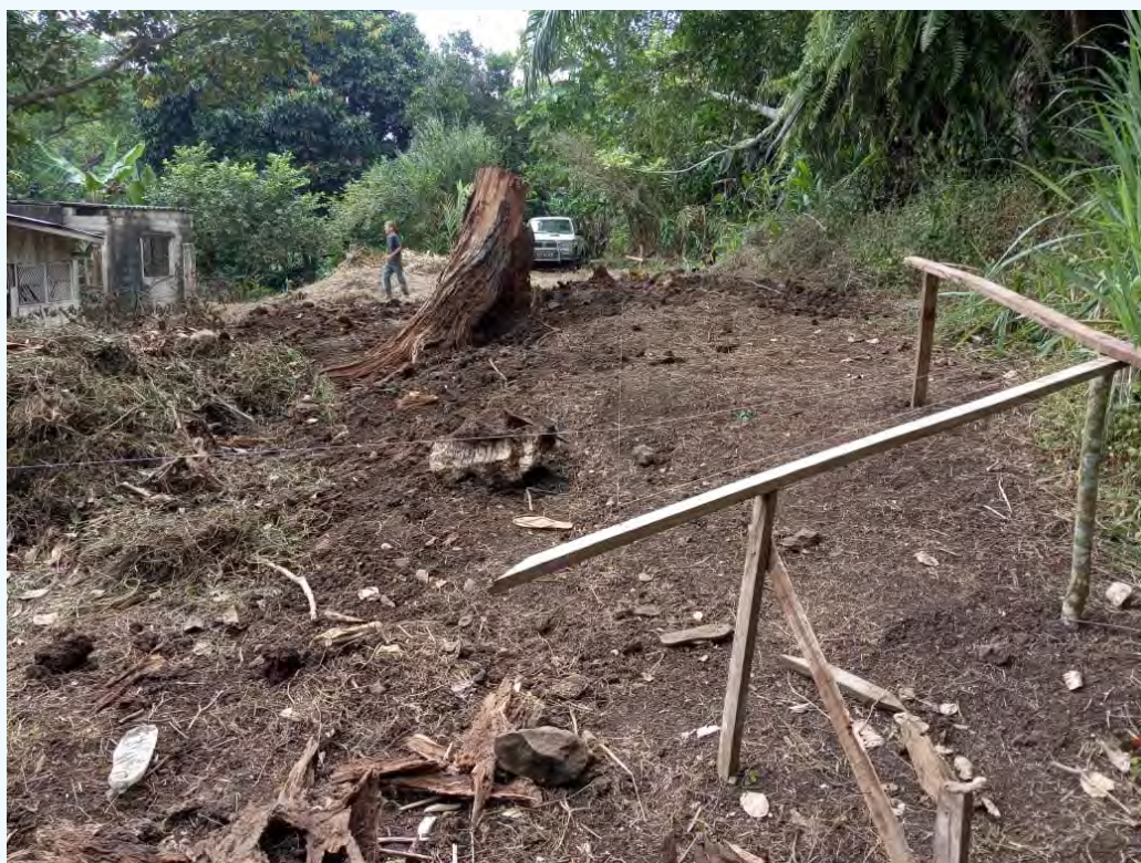
Clearing Ground And Squaring Off The Position Of The House With Fishing Line
