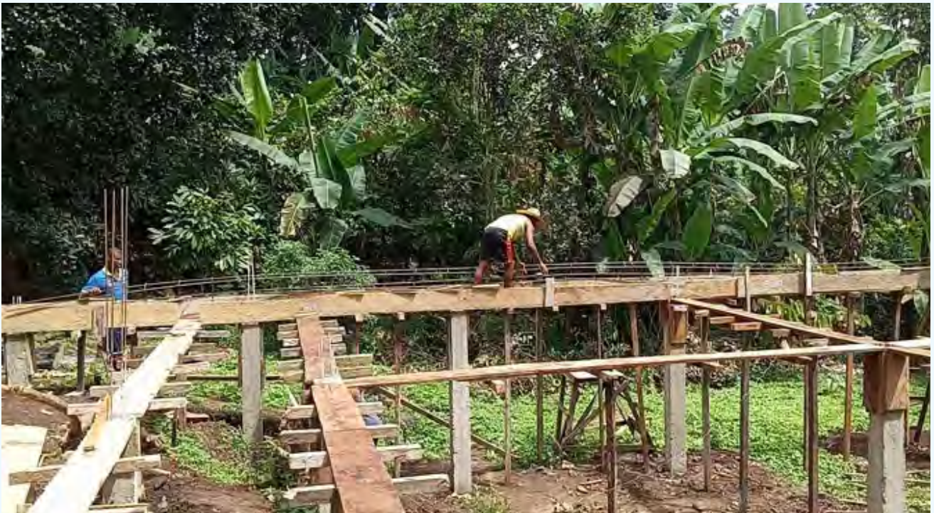
Dropping In The Iron Reinforcements for the Concrete Structural Beams
