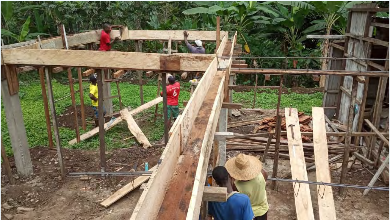
Building Boxes (above) and Tieing Together Iron Reinforcements (below) For The Concrete Structural Beams
