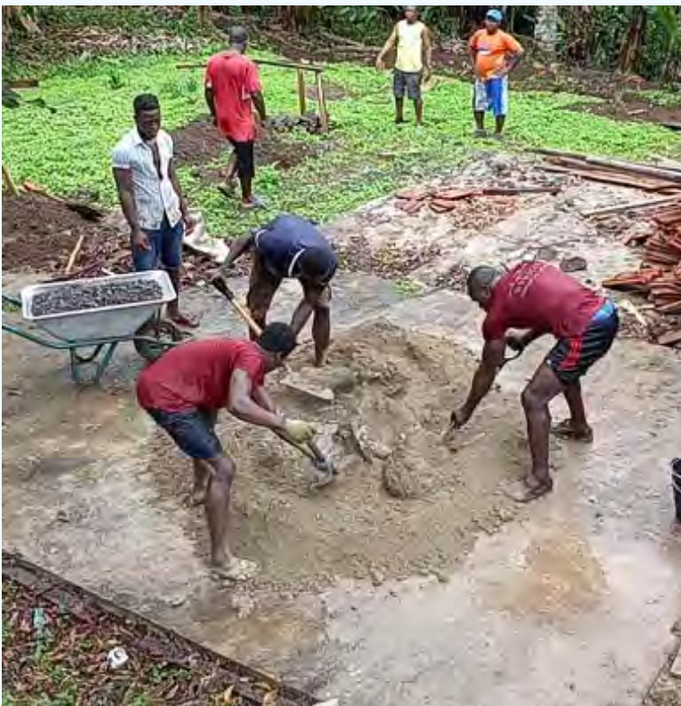
All Of The Concrete Is Mixed By Hand
