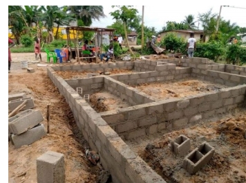
Progress on Ma Bessie's house
