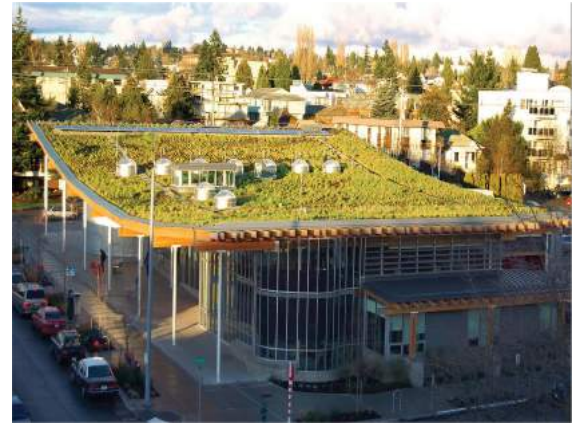
A green roof at Ballard Public Library detains rainwater.
