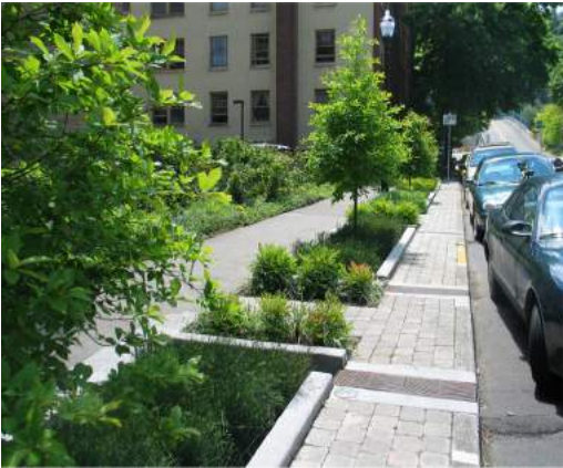
Bioswales on 12th St in Portland detain and clean runoff from paved surfaces.
